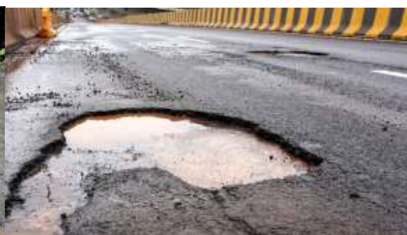
FIGURE 1(b): POTHOLE
