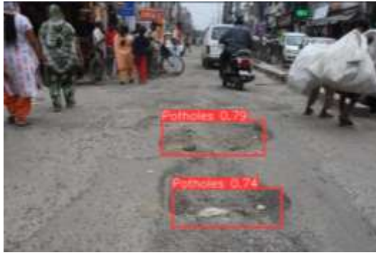
FIGURE 3(a): MULTI POTHOLE DETECTION
